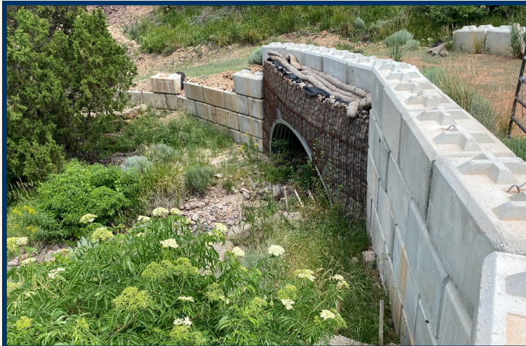
An Aquatic Organism Passage constructed by Newcrest Resources Inc. to protect Bull Trout habitat within the exploration boundary, Elko Co., Aug. 2023.
